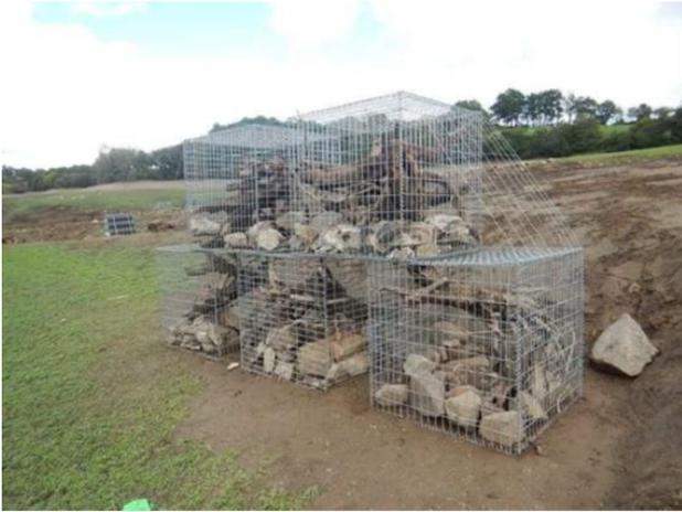
PHOTOGRAPHIE 4 : EXEMPLE DE STRUCTURE TYPE GABION IMMERGEE DANS UN LAC (POSEE ICI A LA FAVEUR D'UNE MISE EN ASSEC)
